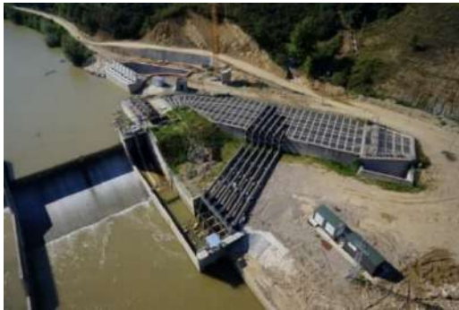
Fig 3. Melen Dam basin Source: [Inc., 2019]
